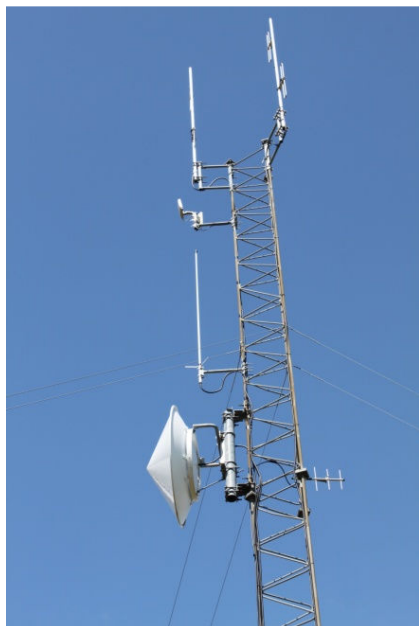
Figure 5-11: Ely Park Tower
