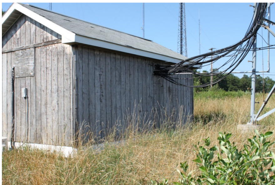
Figure 5-8: Old State Road Site
