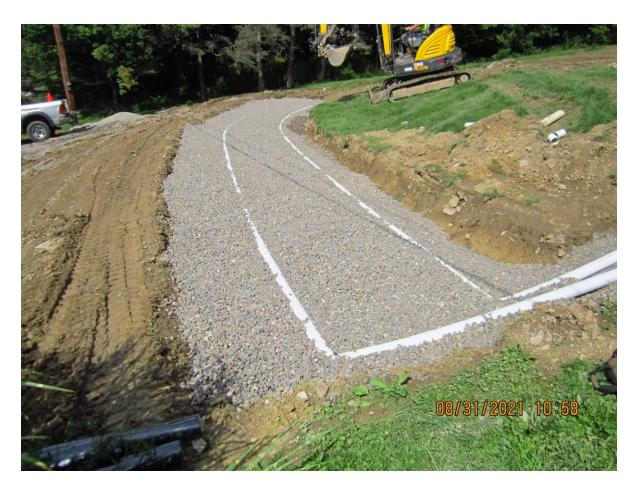
A properly installed modified absorption bed on a slope. Length of bed parallels the site contours, bending to match the gradient. Same depth achieved across length of bed.
