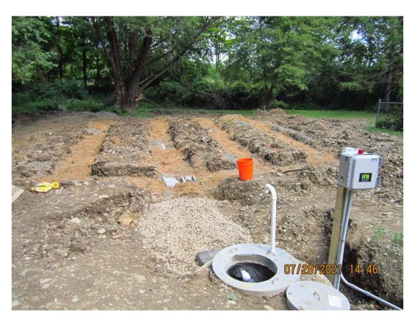
Pump chamber installed to raise effluent exiting septic tank at 4ft depth to trench system installed in shallower useable soil on a flat parcel. See proper venting assembly and pump alarm installed near tank.
