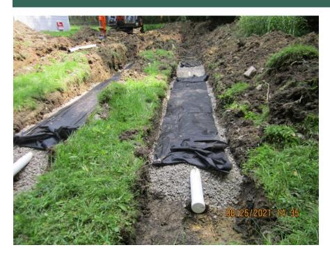
Improperly installed absorption trenches. Trenches running perpendicular to site contours. Deeper at front of trench, shallow at distal end. Trench and bed lengths must run parallel with site contours.
