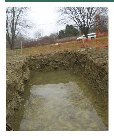
Sand Filter with ground water intrusion. Curtain drain required.
