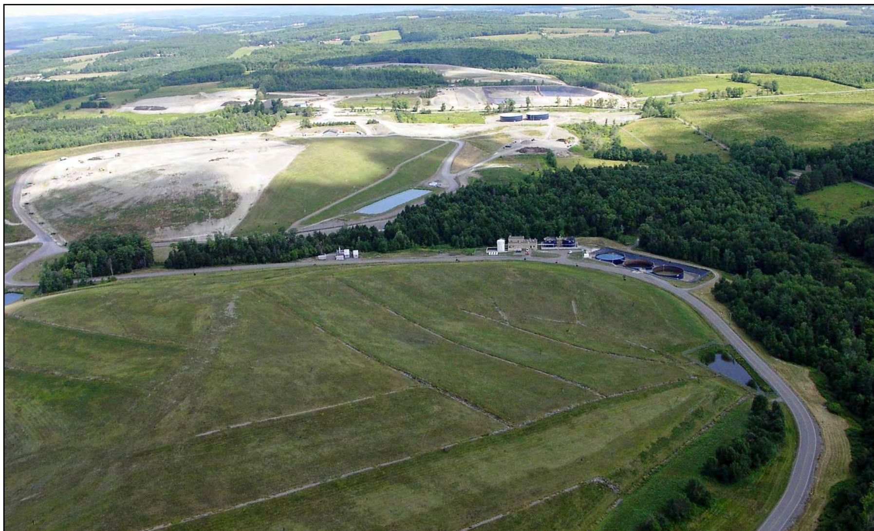
FIGURE 4-2 AERIAL PHOTOGRAPH OF BROOME COUNTY LANDFILL (2002)
